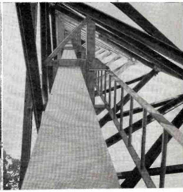
Note sturdy angle supports for both wave guide and ladder.
